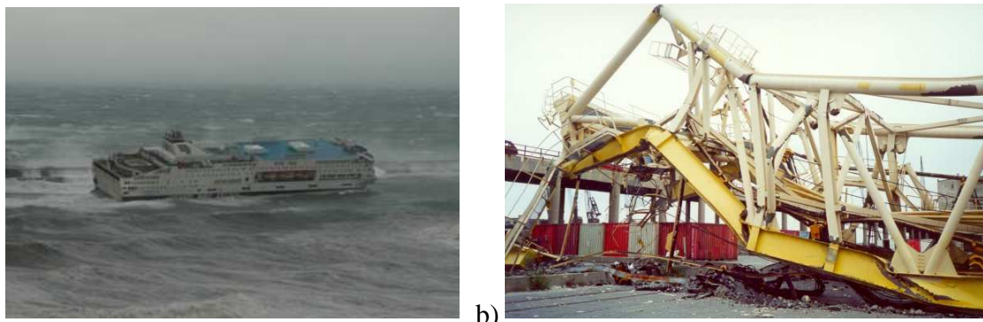
Figure 1. Examples of wind-induced risk and damages in port areas: a) ferry boats coming in Genoa Port; b) collapse of a harbor crane.
