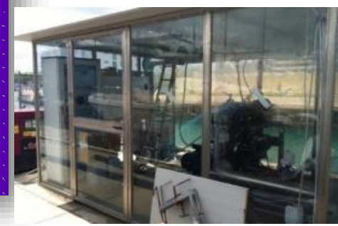
Control room of the ejectors
