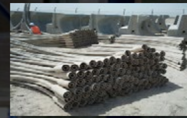
Open Yard Steelworks storage
