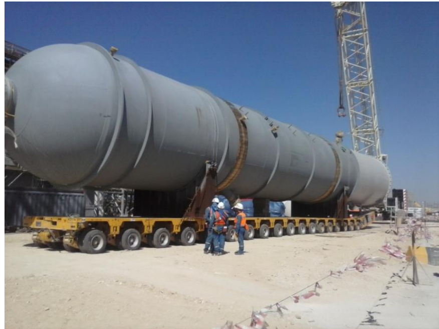
MSPM with HDS Reactor positioned near lifting area for installation at site
