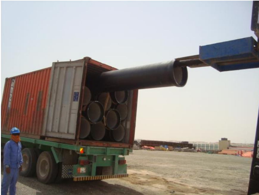
DI pipes being loaded into container
