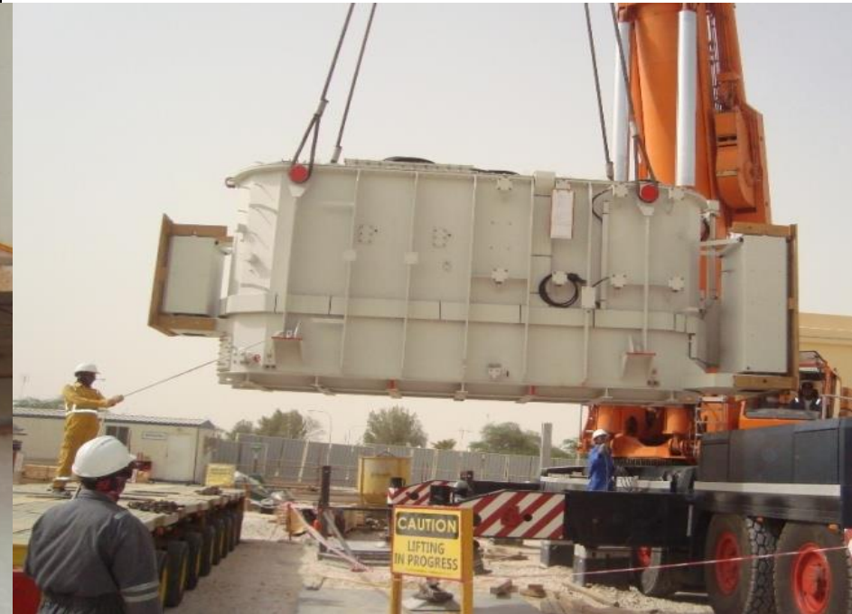
Lifting power transformer from trailer by mobile crane
