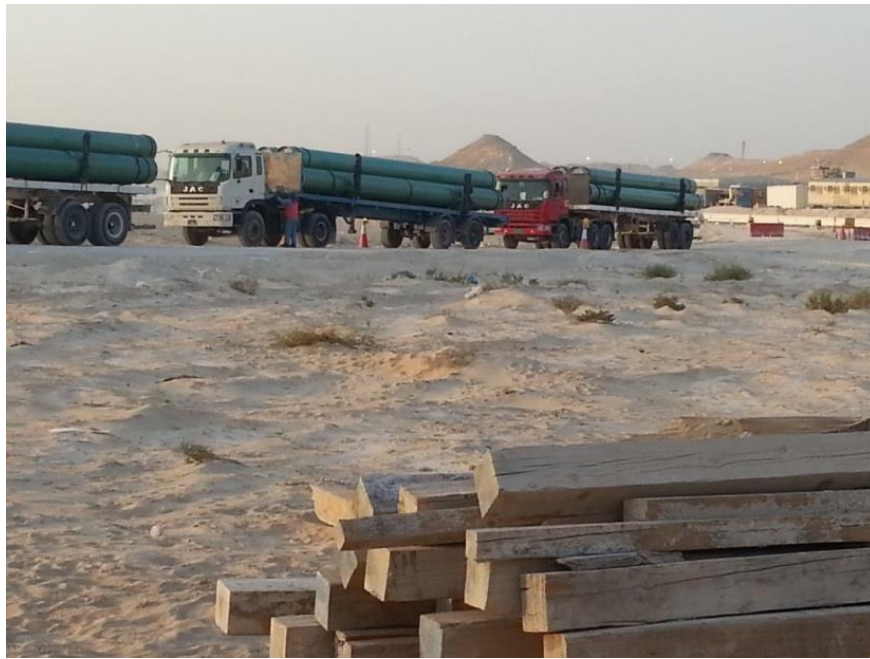
Trailers with gas pipes on steel cradles lined up outside laydown site in Dukhan for unloading
