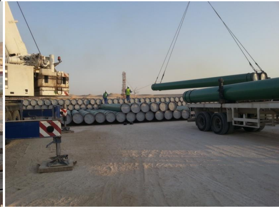
Being unloaded by crane using teflon coated pipe hooks
