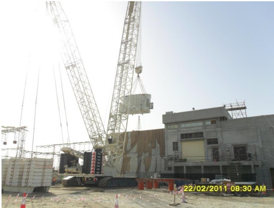
Installation of power transformer on foundation by crawler crane
