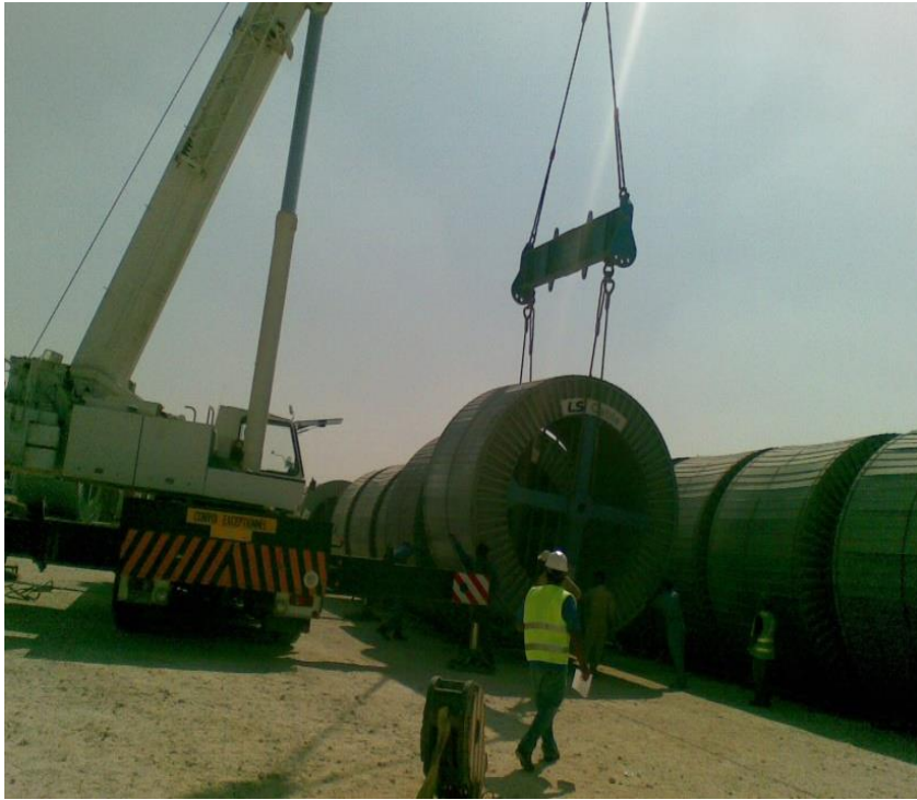
Unloading at site.
