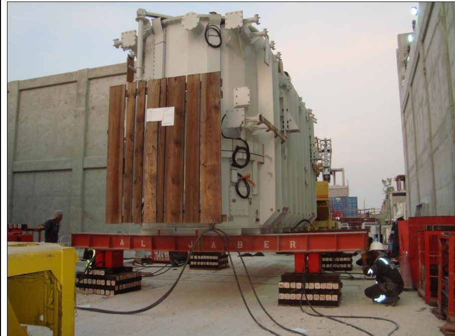
Transformer on beams kept on hydraulic jacks for installation by jacking and skidding process.
