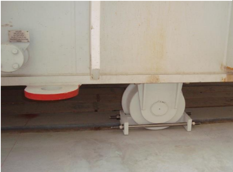
Locking of transformer wheel on the center line of the foundation by nuts and bolts.
