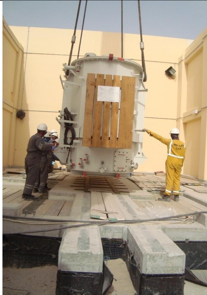
Installation of power transformer on foundation by mobile crane
