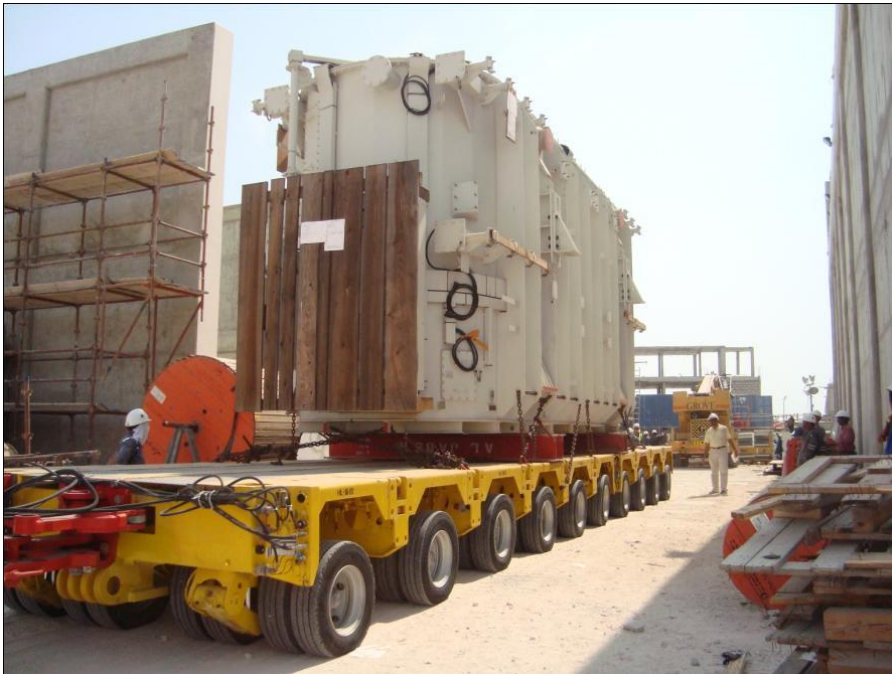
180 ton power transformer being taken into substation site on hydraulic multi axle trailer.
