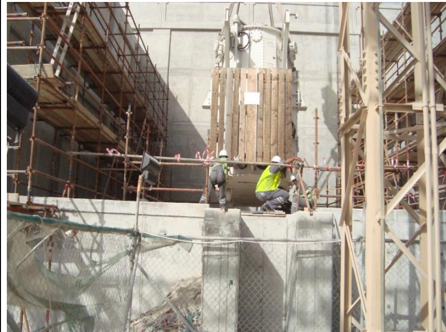
Setting of transformer on foundation.
